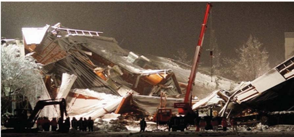
Figure 6-44 – Roof collapse of the Bad Reichenhall ice-arena in 2006 in Germany (from https://www.cbsnews.com/pictures/germany-roof-collapse/18/ )
