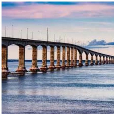
Figure 8-14 – The Confederation Bridge (Canada). (images from https://www.atlasobscura.com/places/confederation-bridge )
