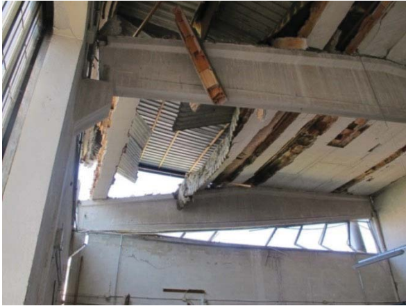
Figure 6-17 – Collapses due to the loss of support of main beams from the column corbel
