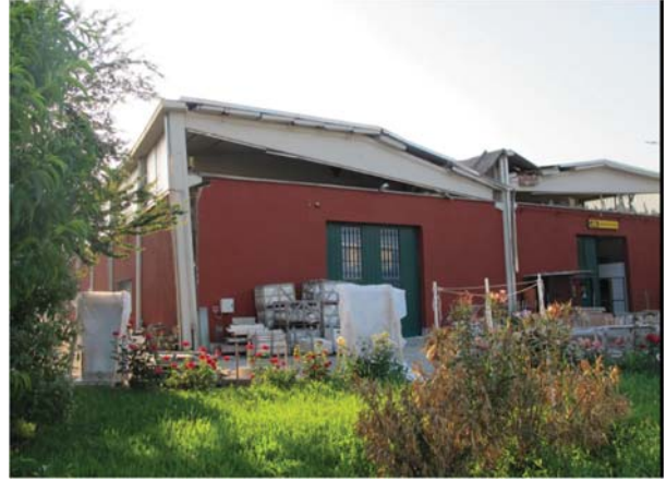
Figure 6-17 – Collapses due to the loss of support of main beams from the column corbel
