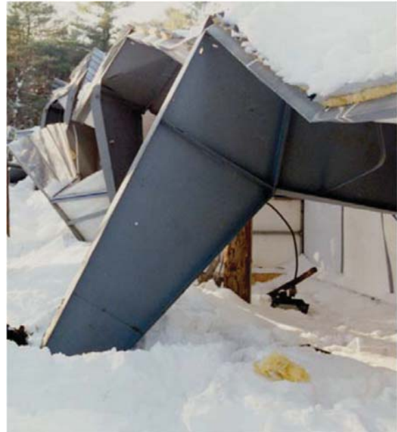
Figure 6-34 – a) details of the structure of the Jackson Landing Skating Rink; b) collapse of the transverse frames (Ellingwood et al., 2007)
