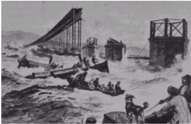
Figure 8-3 – Collapse of the railway Tay bridge (UK) in 1879
