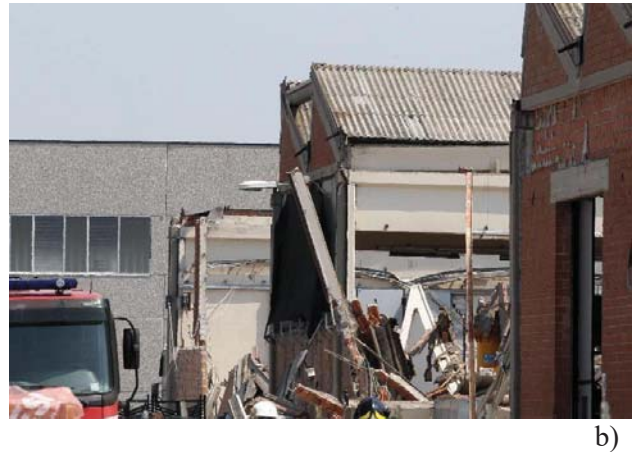
Figure 6-19 – Lateral overturning of high beams with insufficient lateral constraints; a) lateral overturning of plane roof beams with collapse of the upper fork of the columns; b) collapse due to lateral overturning of shed beams
