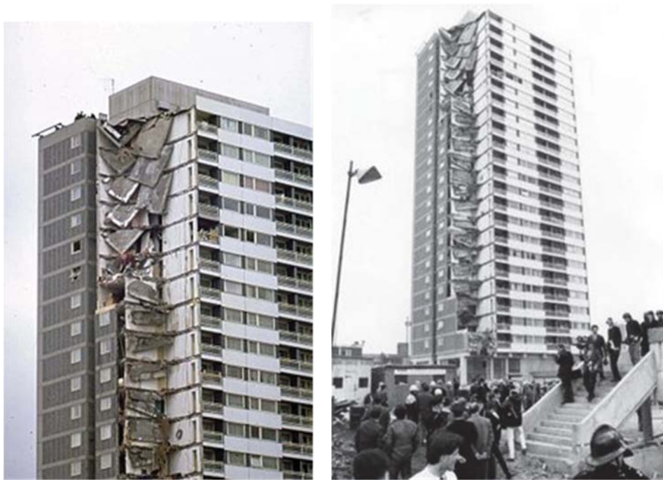
Figure 6-15 – Progressive collapse of a corner portion of a building realized with precast panels (Ronan Point, East London) (from https://en.wikipedia.org/wiki/Ronan_Point )
