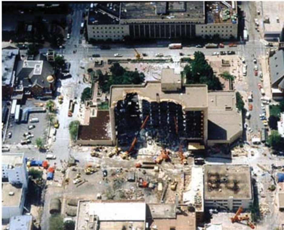
Figure 6-2 – Aerial view after the collapse of the building and the glass facade on the north side (from https://commons.wikimedia.org/wiki/File:Murrah_Building_-_Aerial.jpg )
