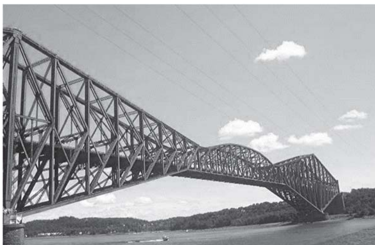
Figure 8-4 – Quebec bridge on the San Lorenzo River in Canada
