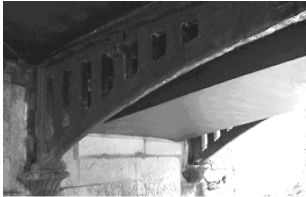
Figure 9-3 – Arch of Corona Bridge after the FRP strengthening.
