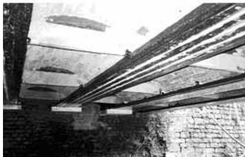
Figure 9-1 – Hythe Bridge (England).
