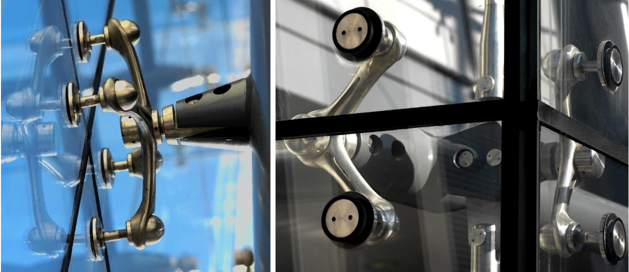
Figure 8.24. Details of Planar type fixing with “spider” supports.
